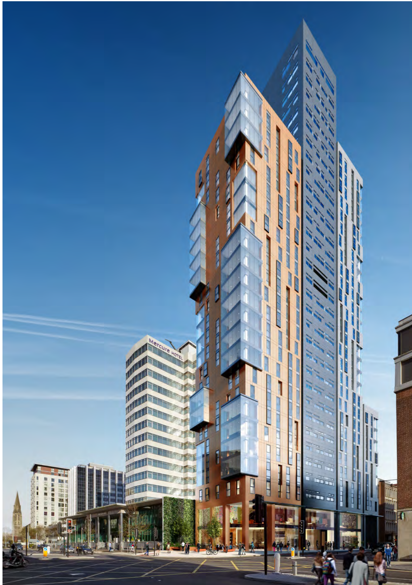
View from Newport Road
